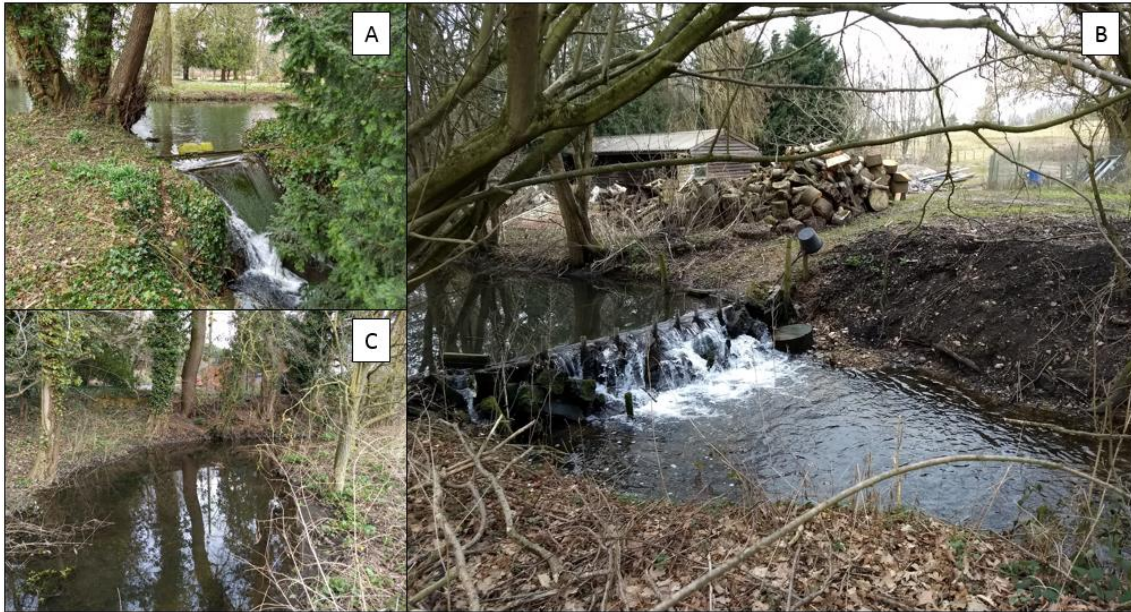
Caption 3.3 Photos of weirs on the surveyed reach of Cantley Stream. (A) Shows the man-made upstream weir (Cantley Stream Pond); (B) Shows a man-made weir upstream of the A47 culvert, (C) Shows water ponding behind the naturally formed weir just east of Cantley Lane South.
